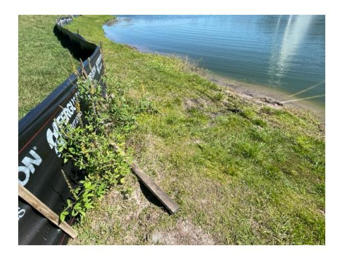
There is a wash-out on the pond bank behind the pool fence. This should be under warranty. The weeds next to the silt fence need to be removed.
