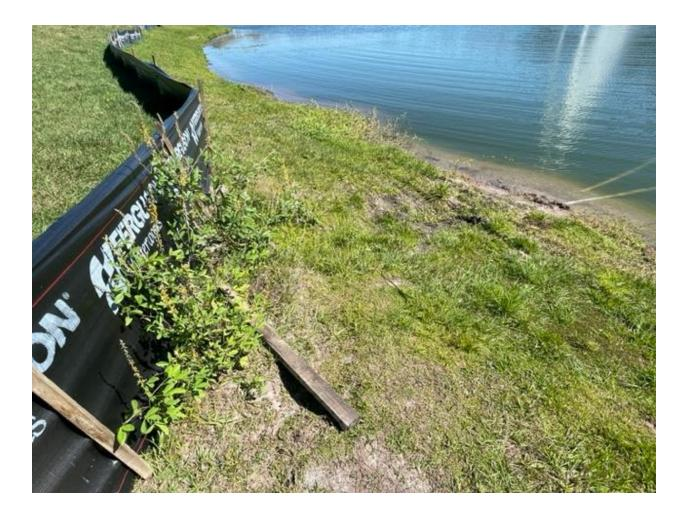
There is a wash-out on the pond bank behind the pool fence. This should be under warranty. The weeds next to the silt fence need to be removed.
